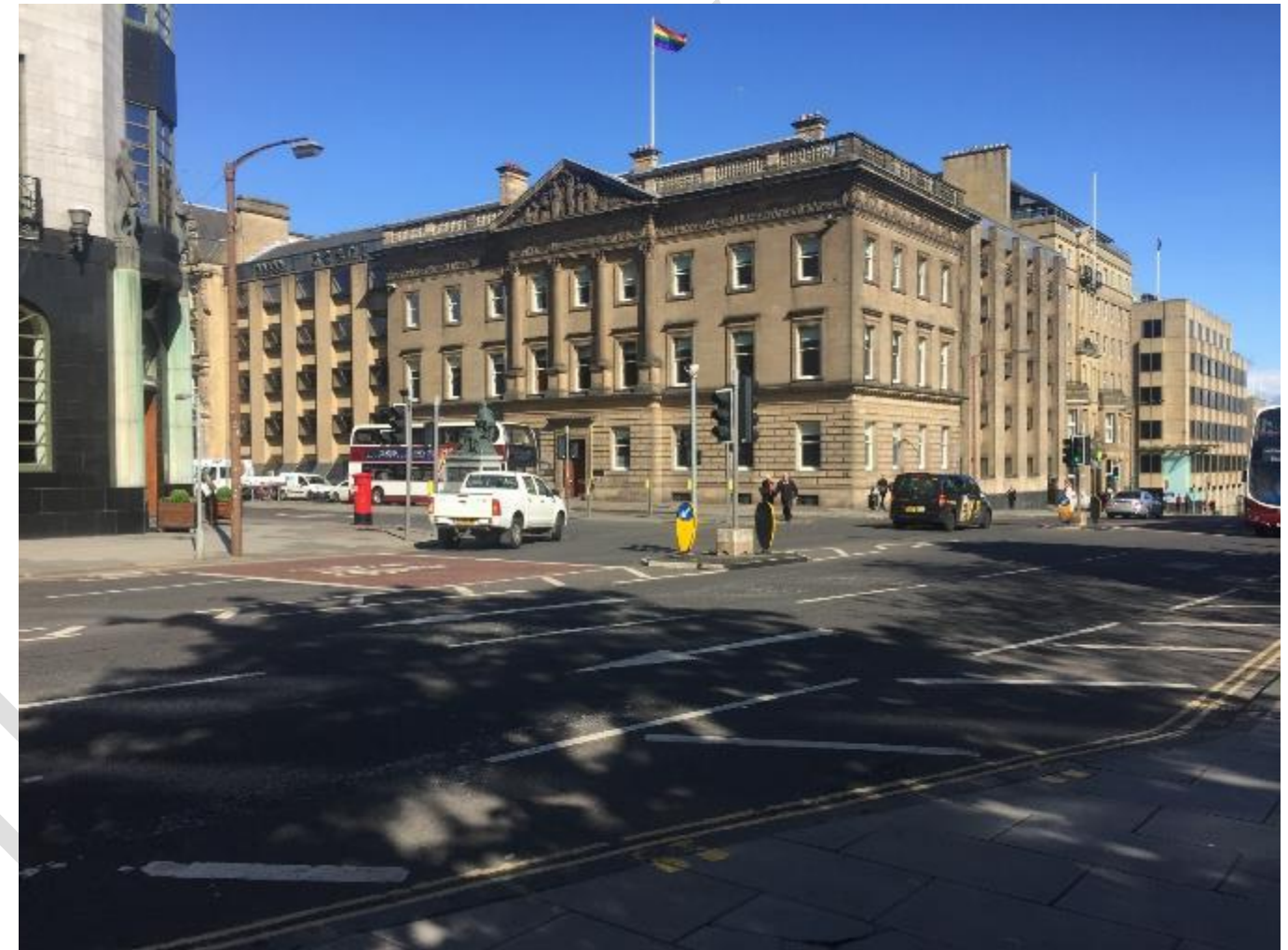
Signalised priority junction of George Street-St Andrews Square
